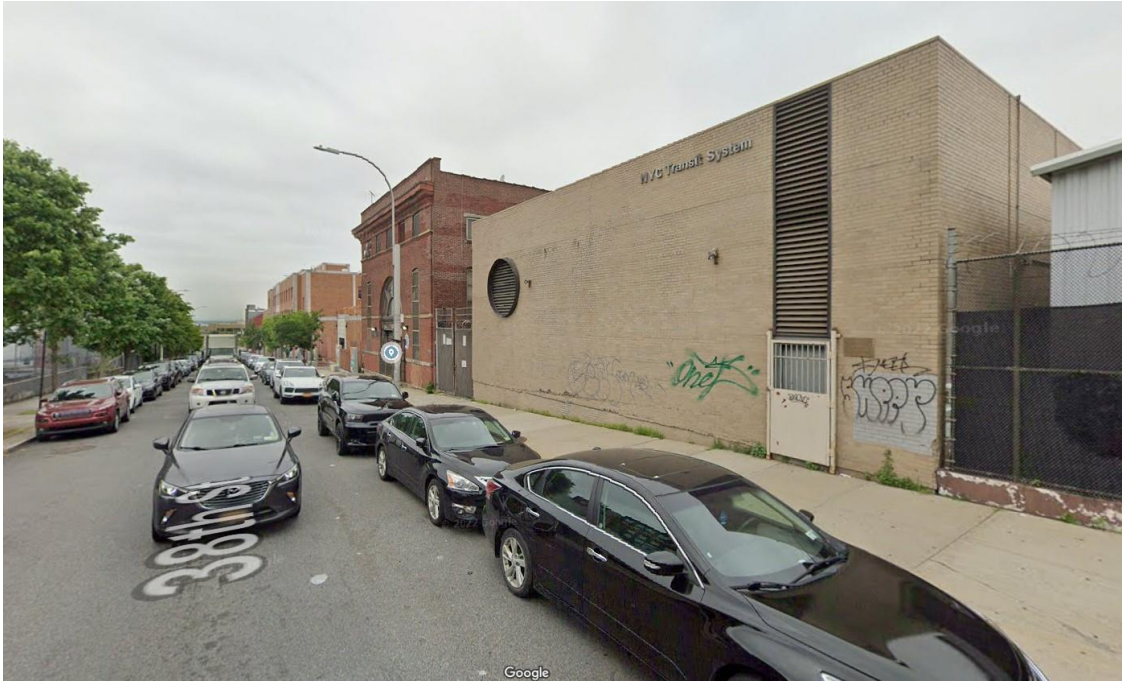
View looking south on 38 th St
