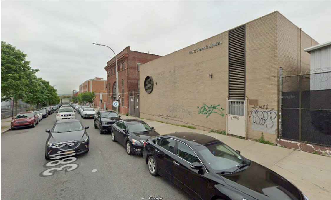
View looking south on 38 th St
