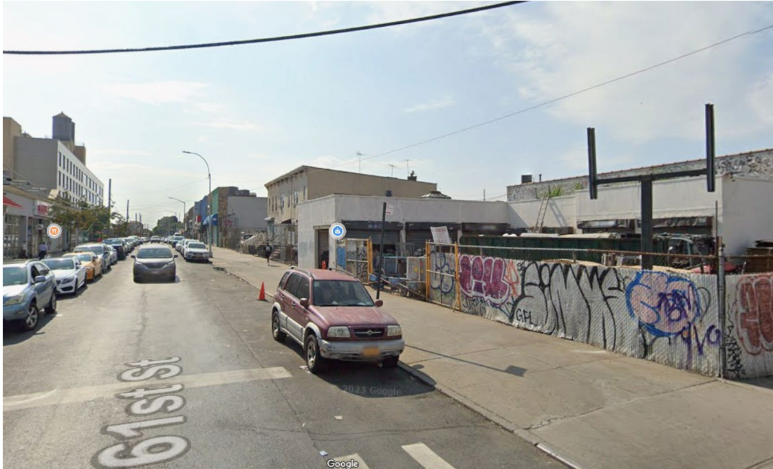
View looking south on 61 st St
